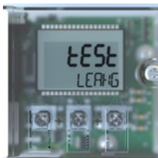
Leak Test Initiated
